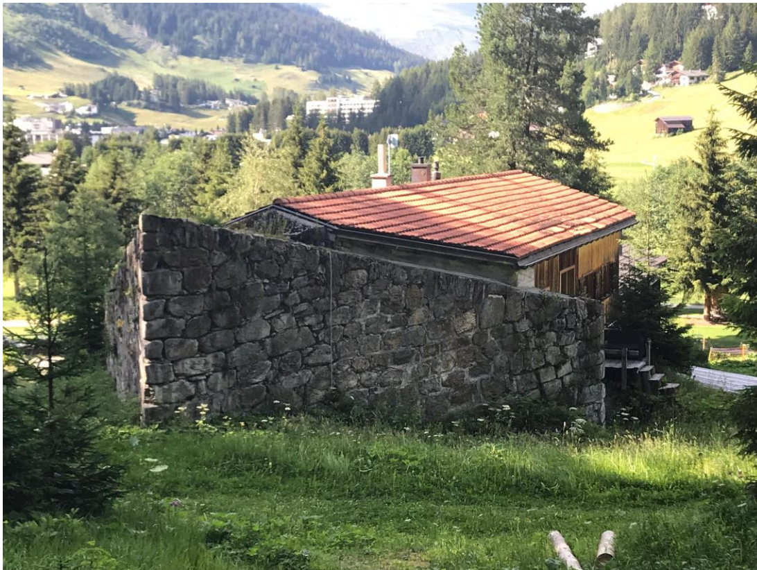
Figure 6.34: A symmetric splitting wedge protecting a house near Davos. The cutting angle of the wedge is approximately 2\alpha_2 = 60^\circ .
